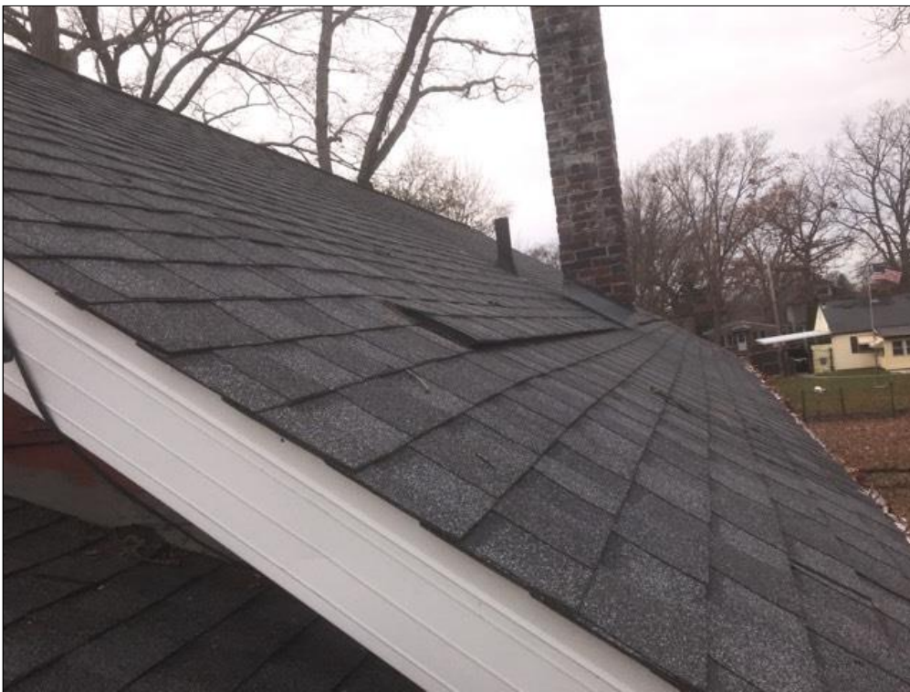
1.0 Item 1(Picture) roof overview
