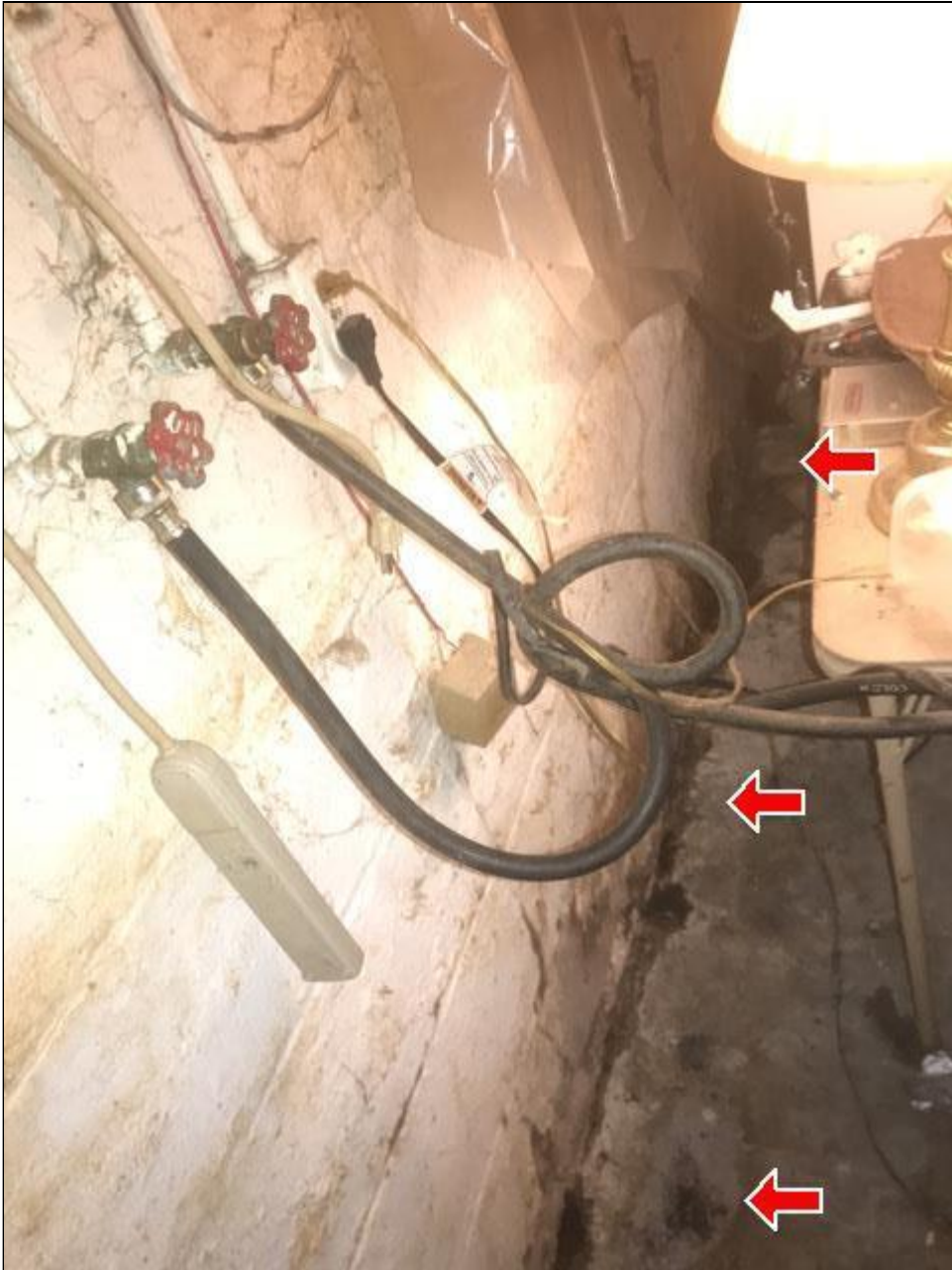
5.0 Item 2(Picture) basement north perimeter
