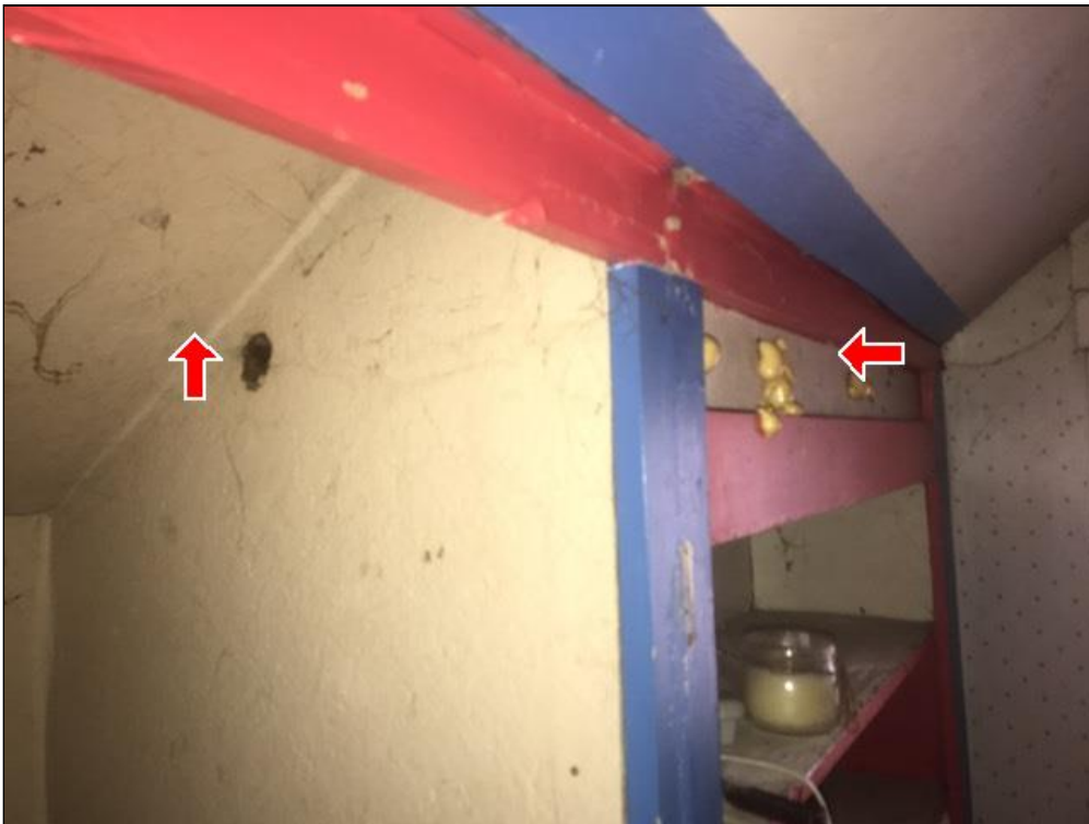
5.5 Item 2(Picture) attic ceiling
