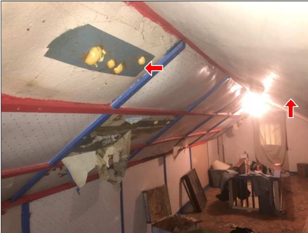
5.5 Item 1(Picture) attic ceiling
