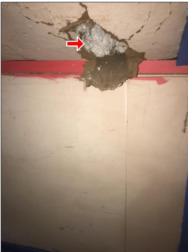
5.5 Item 3(Picture) attic ceiling insulation
