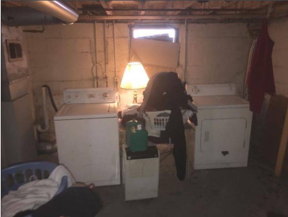
5.0 Item 1(Picture) basement water intrusion area
